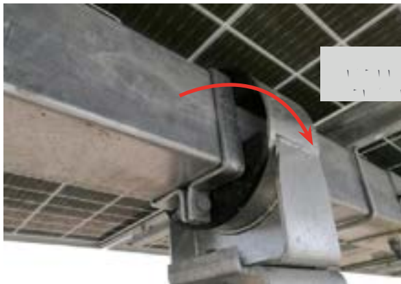
1 Cylindrical bearing structure
